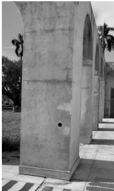
Concrete core samples taken from 14 locations were tested to determine the strength of walls and columns.
